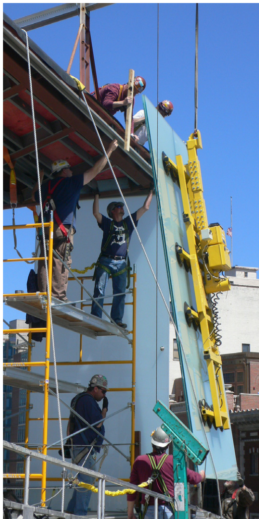
LANTERN GLASS INSTALLATION
